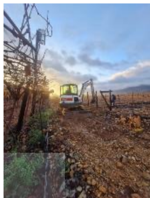
Right: Excavation equipment preparing the soil for planting.
