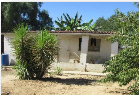
Staff houses before renovation:
