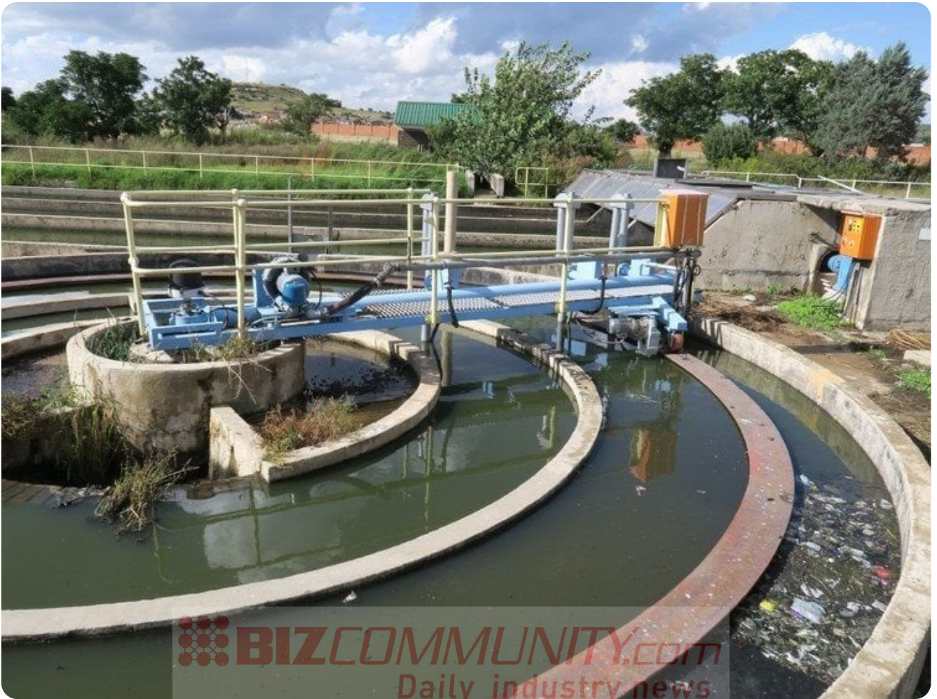
A dysfunctional sewage treatment works in Winburg, Free State, from which sewage flows untreated into the dam from which drinking water for the town is extracted.
