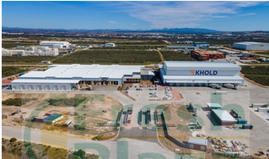
Under one roof: a citrus packhouse, cold store and container depot (photo supplied by KHOLD)
