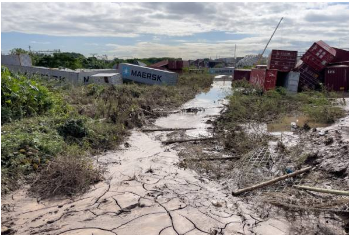
Flood damage in Durban, South Africa, in 2022 | Archive
