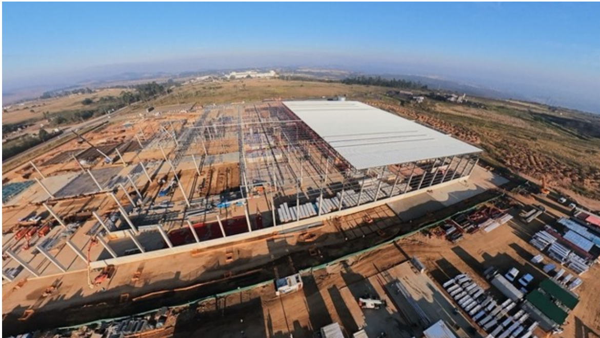
© FPT Group FPT cold rooms under construction in Cato Ridge, a back-of-port facility to Durban port
