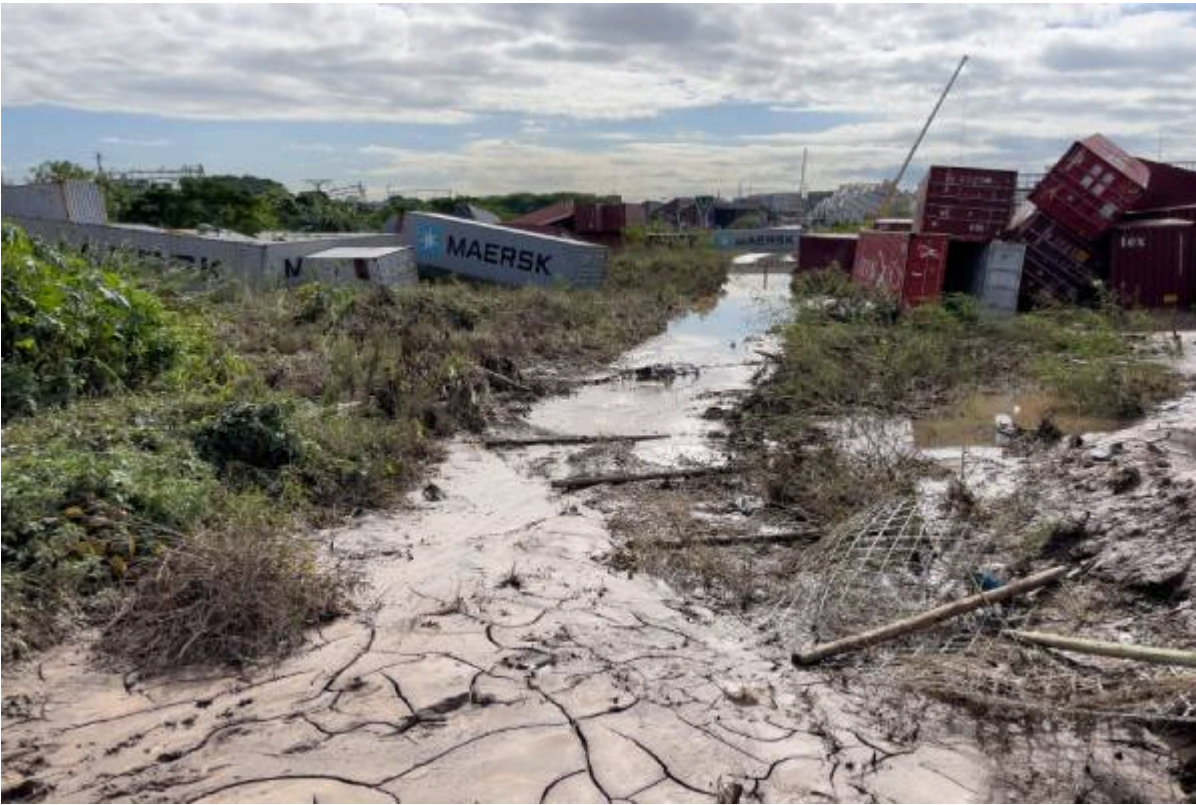
Flood damage in Durban, South Africa, in 2022.
