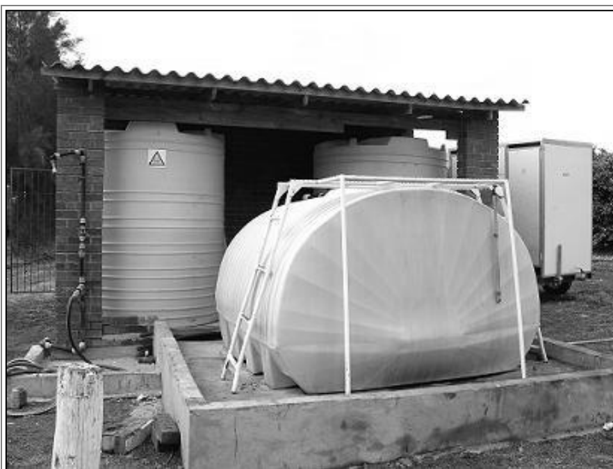
Fertigation Tanks
