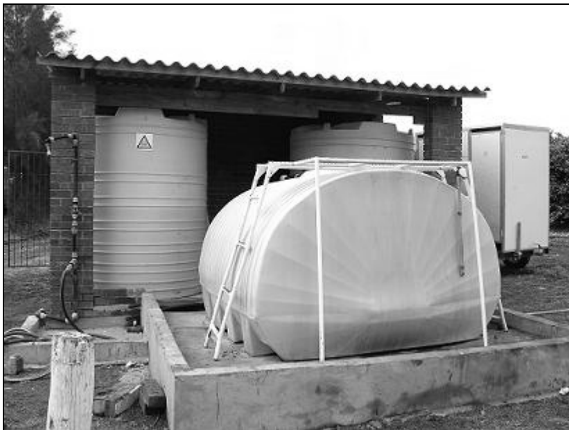
Figure 4.1: Fertigation Tanks at Crookes Brothers (Nkwalini)
