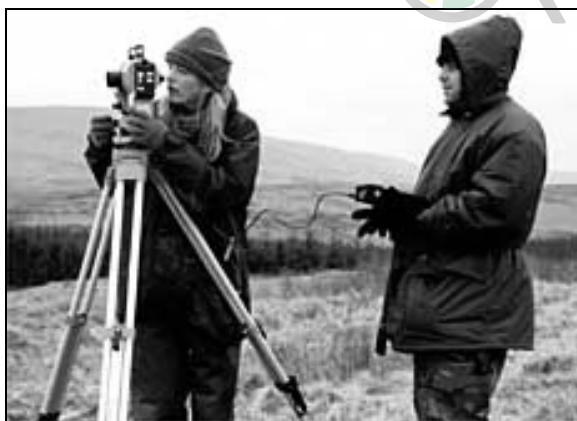
Figure 2.1: Using a Theodolite to Lay Out a New Orchard
