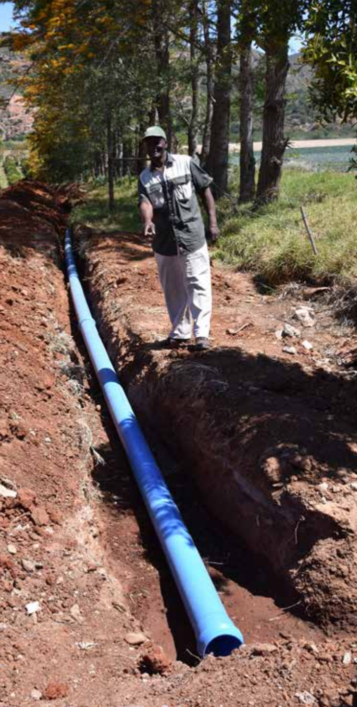
Jack Peter shows the progress with the installation of the water supply and irrigation system for the farm's new orchards.
